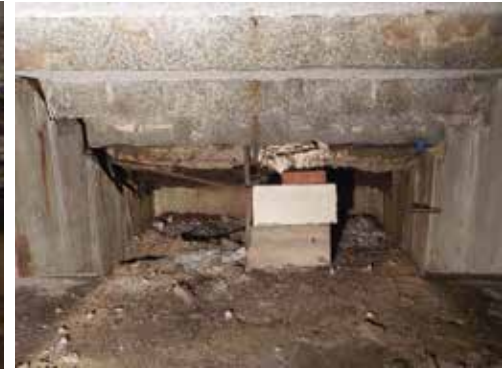
Clockwise from top left: North stair prior to restoration. 1977 precast concrete raker beam structure and circa 2011 retrofit steel shoring. Deteriorated precast raker beam, tread bedding mortar, and concrete plaza slab at north end of stair. Retrofit channels installed beneath broken granite treads.
