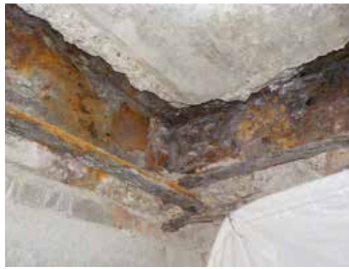
From left to right: Severely corroded existing steel framing beneath the colonnade deck. Replacement colonnade steel structure.
