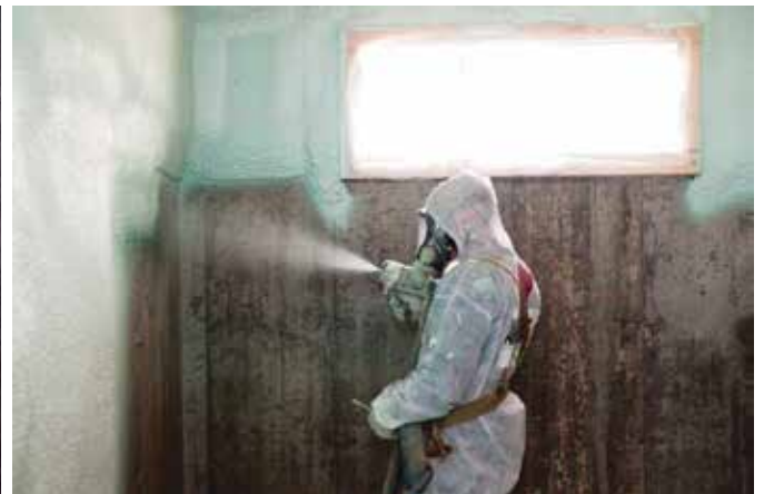
Spray polyurethane foam (SPF) plays a significant role in mitigating common air leakage paths, such as joints, seams, and penetrations, thereby enhancing the airtightness of buildings.
