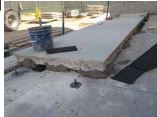
Clockwise from above: Forming and reinforcing steel for new c.i.p. concrete stair structure. Two-ply waterproofing membrane on top of concrete stair structure. Granite landing stones laid on grout pads complete with stainless-steel dowels.
