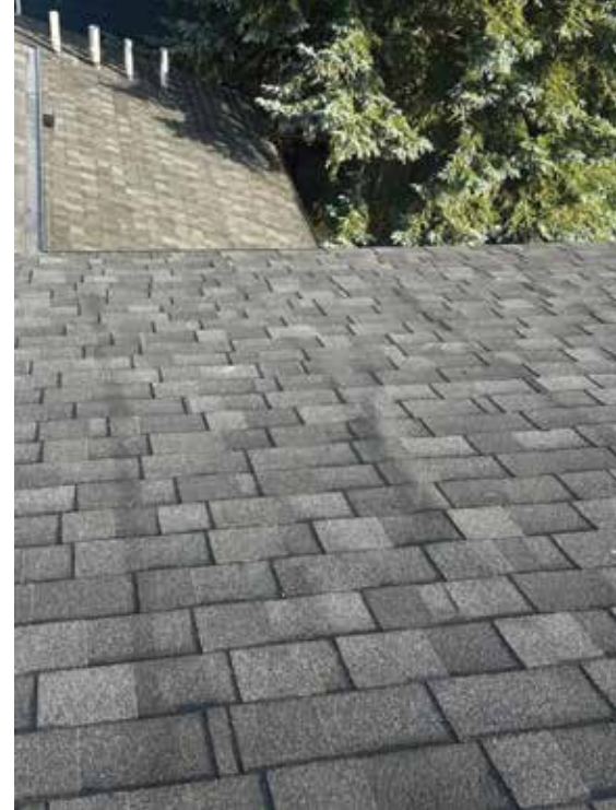
Photo 1 - Steep slope roof, ridging clearly visible in shingles following the rafters.
