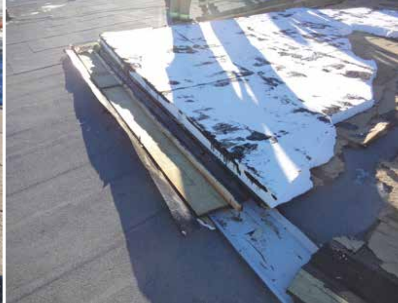
Photo 3 - Underside of roof assembly showing parapet components which had been nailed to the CMU parapet.
