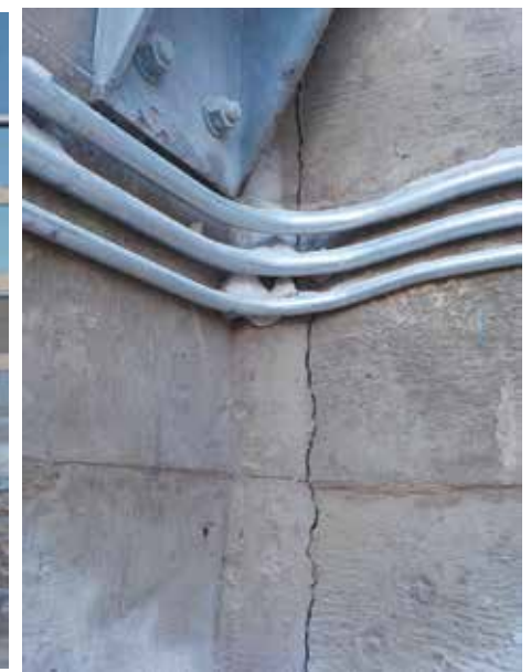
Clockwise from left: Eastern freestanding columns and concrete pilasters. Cracking between concrete north corridor wall and east concrete pilaster. Diagonal cracking with masonry portion of east freestanding column pilaster. Pilaster tie system.
