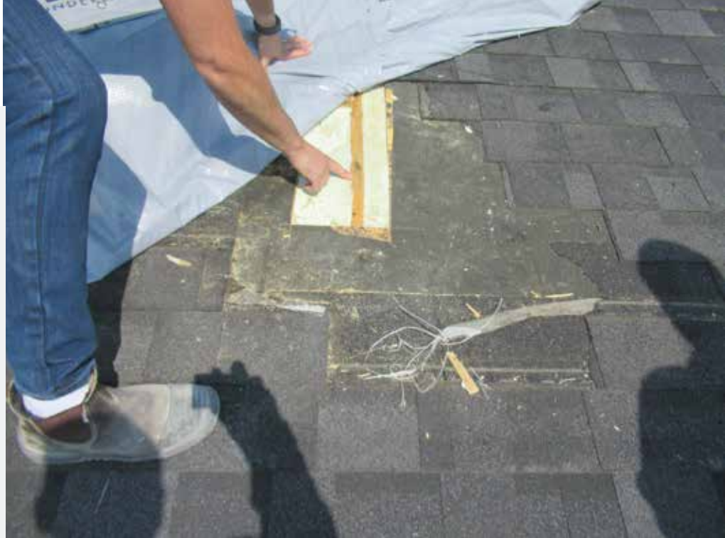
Photo 3 - Roof investigation at one of the shingle ridging locations. Sheathing removed to expose spray foam.
