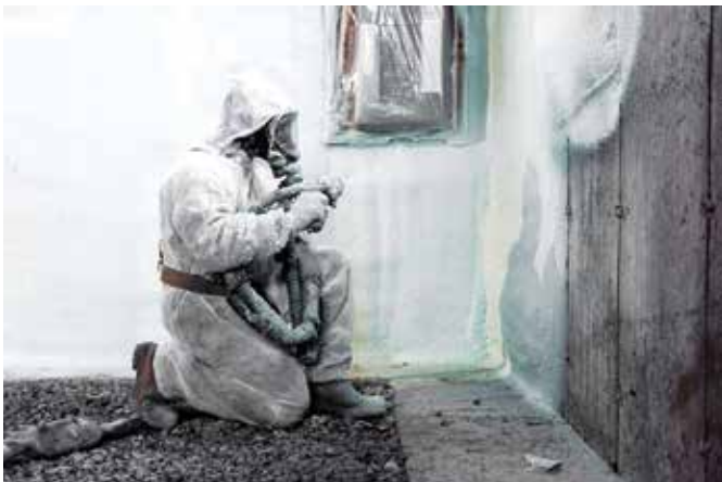
Spray polyurethane foam (SPF) plays a significant role in mitigating common air leakage paths, such as joints, seams, and penetrations, thereby enhancing the airtightness of buildings.
