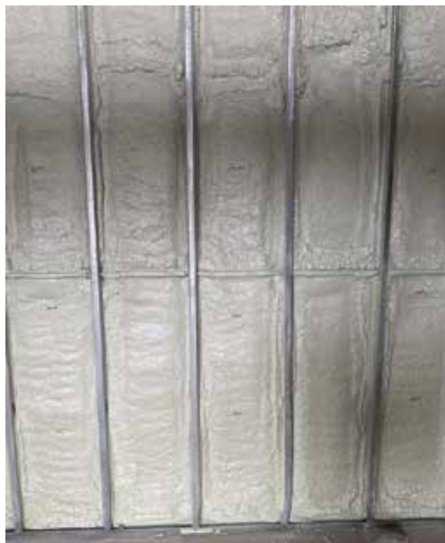
Far left: Application of hydrofluoroolefin (HFO) to achieve high RSI-values.
