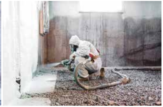
Contractor spraying a polyurethane spray foam insulation product. Photo courtesy Huntsman Building Solutions (HBS).
