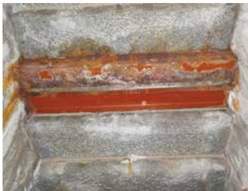
Clockwise from top left: North stair prior to restoration. 1977 precast concrete raker beam structure and circa 2011 retrofit steel shoring. Deteriorated precast raker beam, tread bedding mortar, and concrete plaza slab at north end of stair. Retrofit channels installed beneath broken granite treads.
