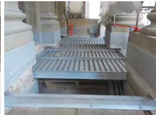
From left to right: Severely corroded existing steel framing beneath the colonnade deck. Replacement colonnade steel structure.
