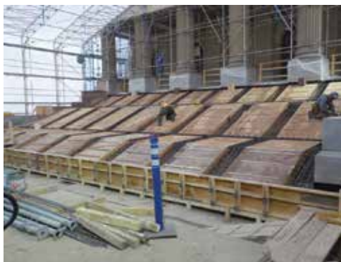
Clockwise from above: Forming and reinforcing steel for new c.i.p. concrete stair structure. Two-ply waterproofing membrane on top of concrete stair structure. Granite landing stones laid on grout pads complete with stainless-steel dowels.
