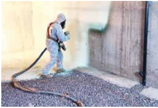
Contractor spraying a polyurethane spray foam insulation product. Photo courtesy Huntsman Building Solutions (HBS).
