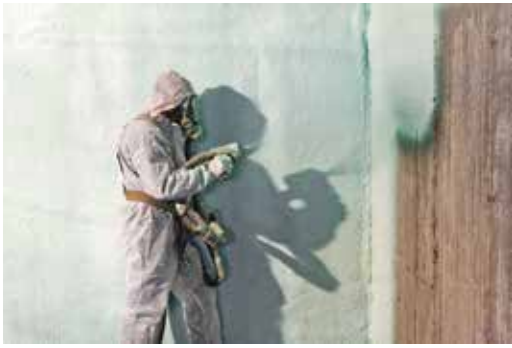
Contractor spraying a polyurethane spray foam insulation product. Photo courtesy Huntsman Building Solutions (HBS).
